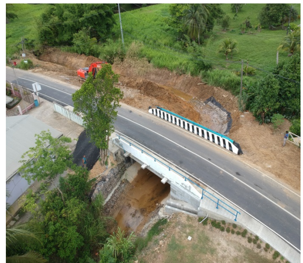
Figure 2. Completed Works on Freeport Todd's Road Bridge
