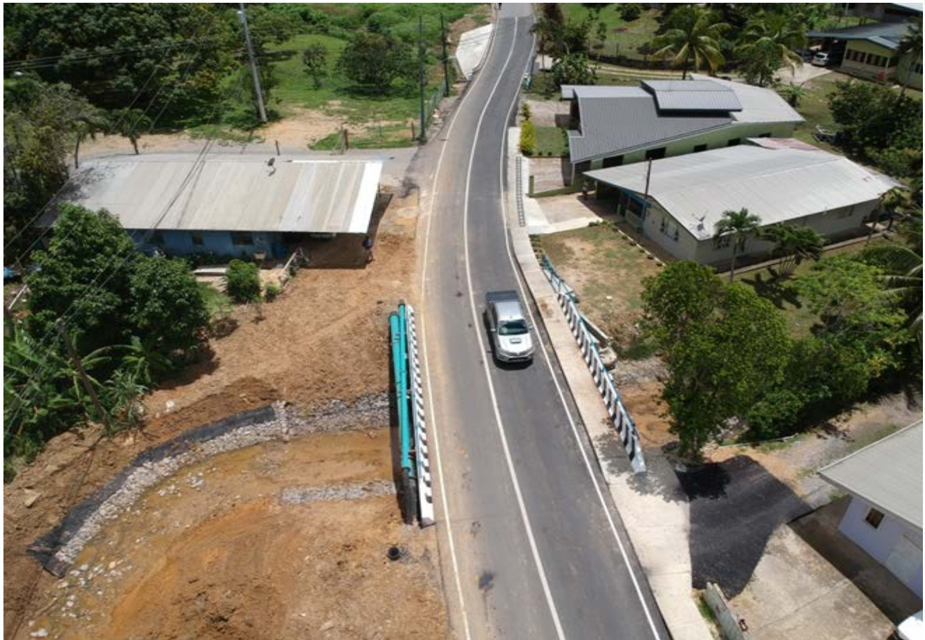
Figure 6. Aerial view Bridge B1/1 Freeport Todd's Road after Construction.
