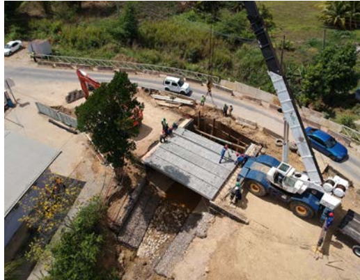
Figure 4. Bridge B1/1 Freeport Todd's Road during Construction.
