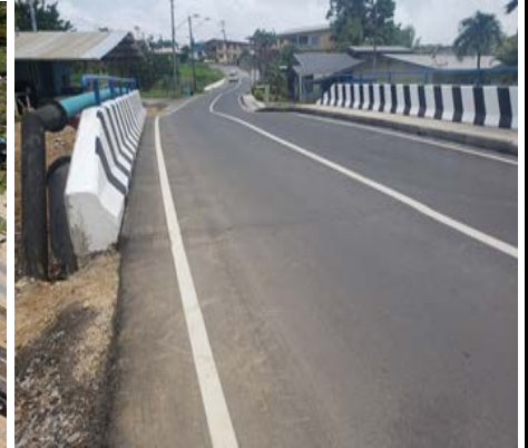
Figure 5. Bridge B1/1 Freeport Todd's Road after Construction.
