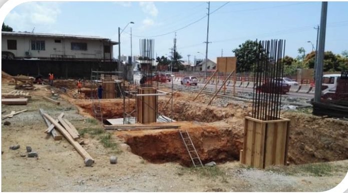
Figure 2 - Beginning stage of Construction
