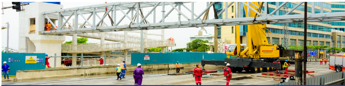
Water Taxi Pedestrian Overpass, Wrightson Road
