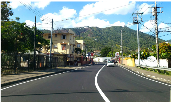
St. Ann's Main Road Rehabilitation
