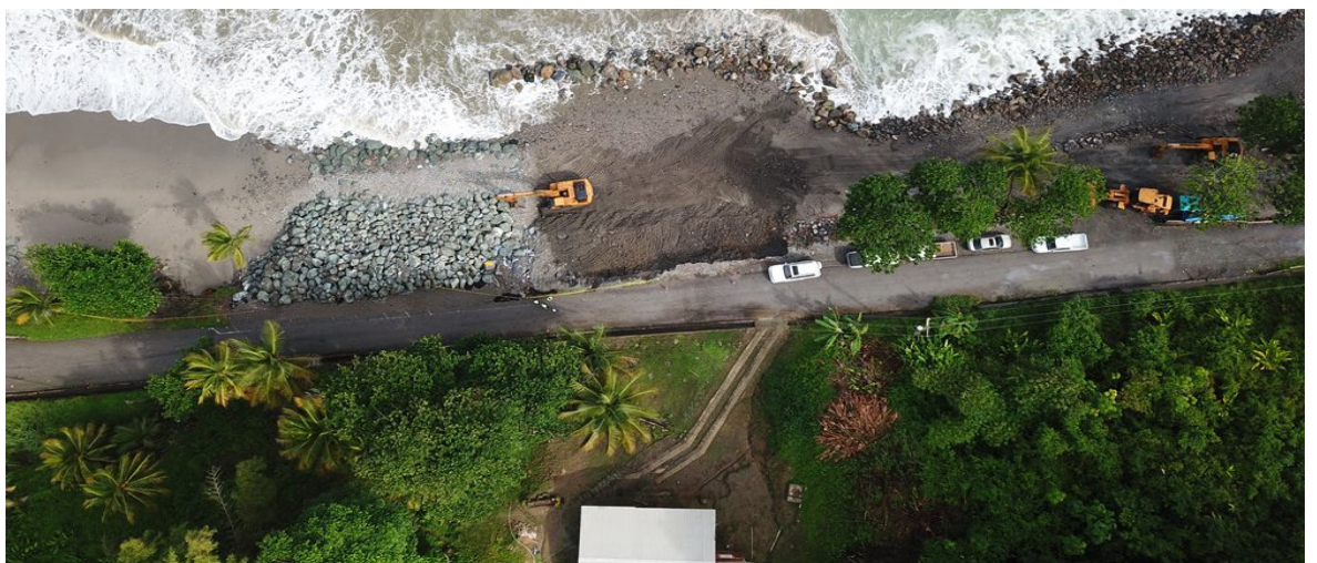
Matelot Shoreline Stabilization Works
