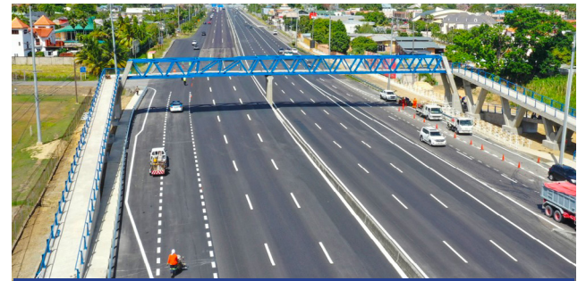
Valsayn Pedestrian Overpass
