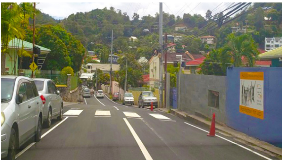
Cascade Main Road Rehabilitation
