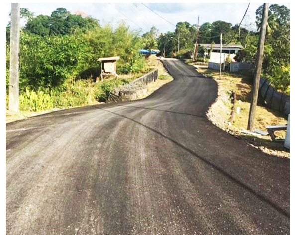
Mundo Nuevo Slope Stabilization
