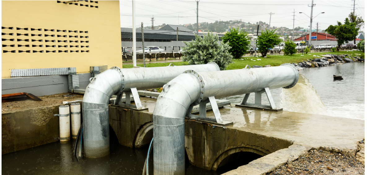
City Gate Pump Site to support the Port of Spain Flood Alleviation Project
