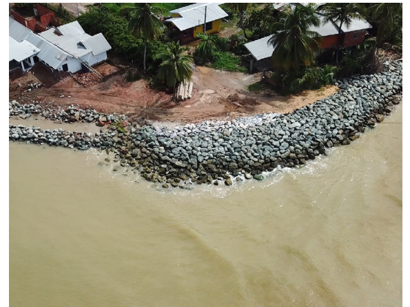
Cap de Ville Shoreline Stabilization Works
