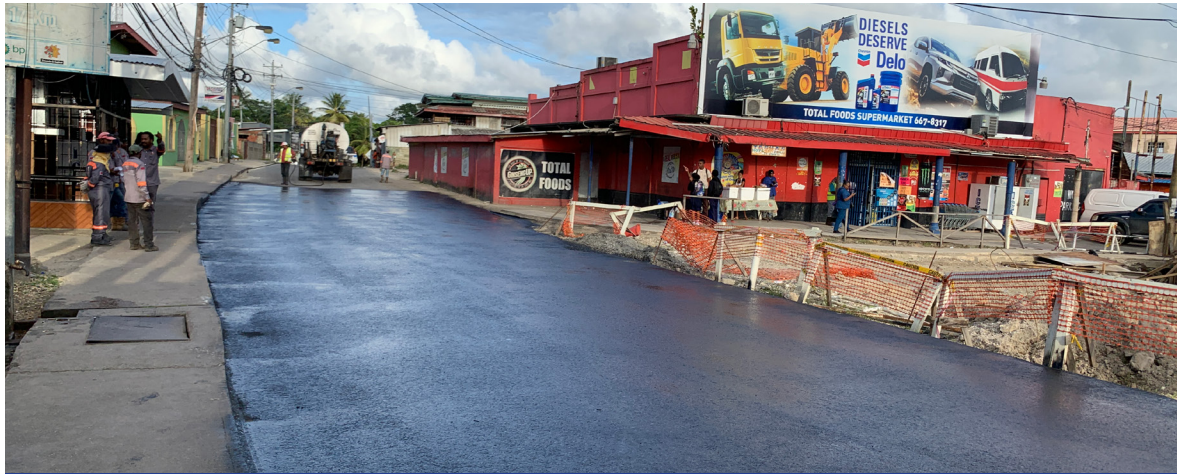
Valencia Road Rehabilitation
