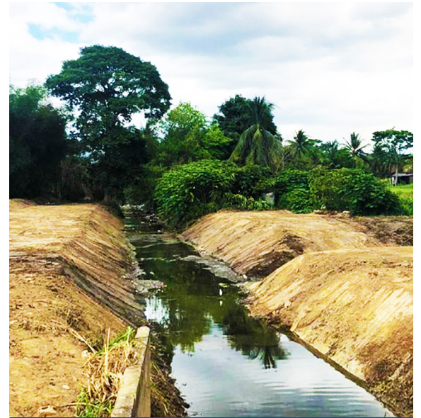
Blackman Ravine Desilting Works
