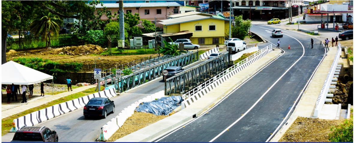
B1 / 35 Bridge Southern Main Road, Cross Crossing San Fernando
