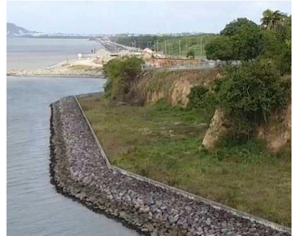
Shore of Peace Cliff Stabilisation Works
