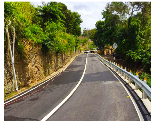
Beau Pres Slip Stabilization
