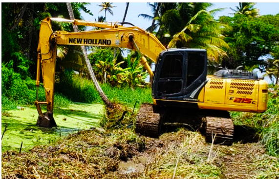
Ocean Sands Drain Desilting Works
