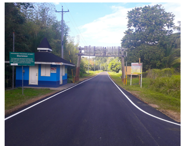
Tucker Valley Road Rehabilitation
