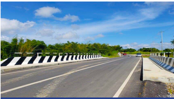
Freeport Mission Road Rehabilitation
