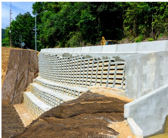
North Coast Road Slope Stabilization
