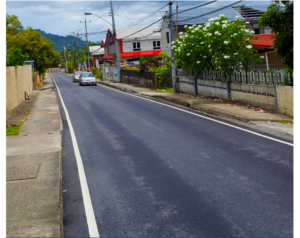
St Lucien Road Rehabilitation Project
